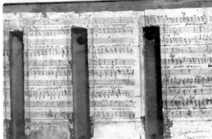
69 Detail of the lower part of the windchest papered with the music score
